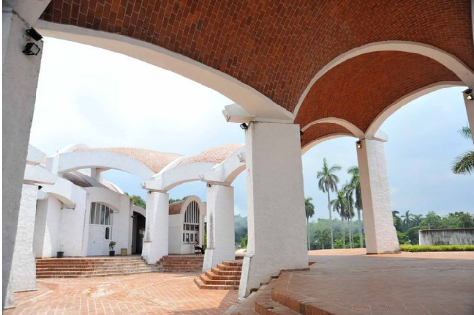
Mr. Porro also designed the School of Modern Dance in Cuba, with brick domes and vaults built by hand in the Catalan style. Credit "Unfinished Spaces" by Alysa Nahmias and Benjamin Murray
